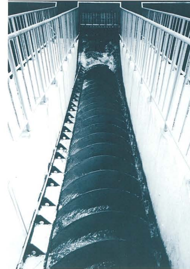
Delivered to the Hiro Pumping Station, Hiroshima pref. Screw dia: 1,300mm.
